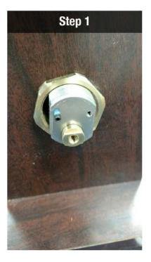
Install cam lock through the drilled hole and use mounting nut to tighten lock intoplace
