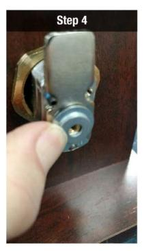
Install the washer on TOP of Rotation Control Plate
